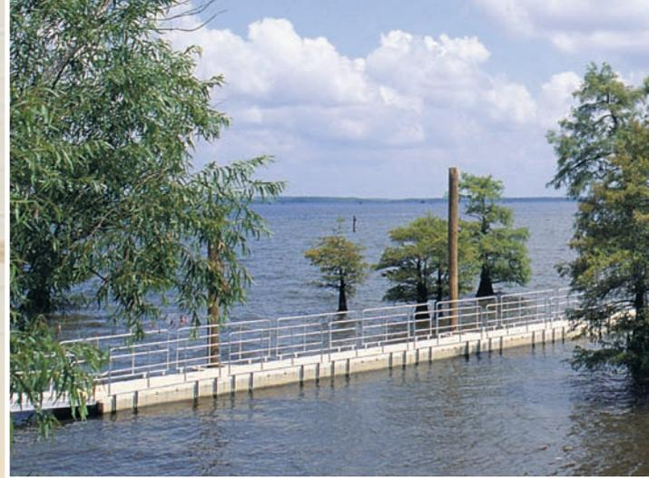
The hollow sections provide stable flotation, and they can be suspended above vegetation during periods of low water, so as not to harm the habitat.
